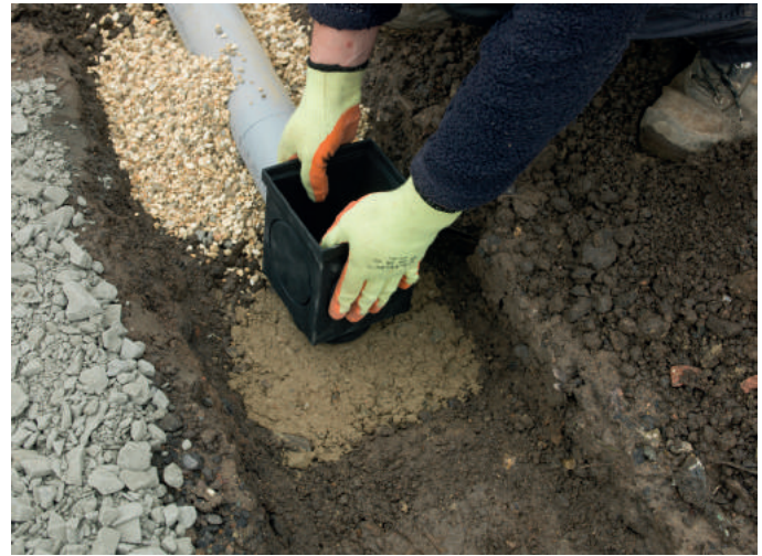
2. Drainer Outfalls and Rodding boxes should be installed first along with relevant pipe work to relevant soakaway or SuDs compliant system.
