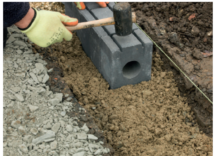
4. Lay the units onto a freshly mixed workable bedding concrete making sure you achieve a tight connection between each unit.
