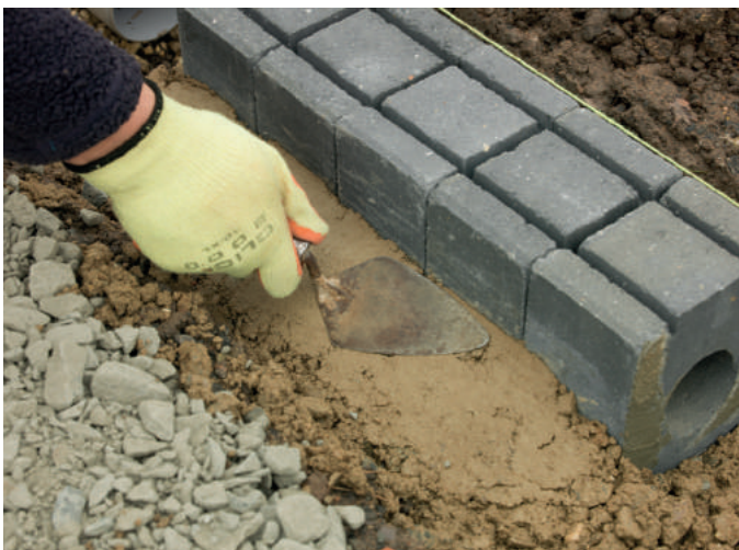
5. Haunch the units using bedding concrete of an appropriate thickness and depth.
