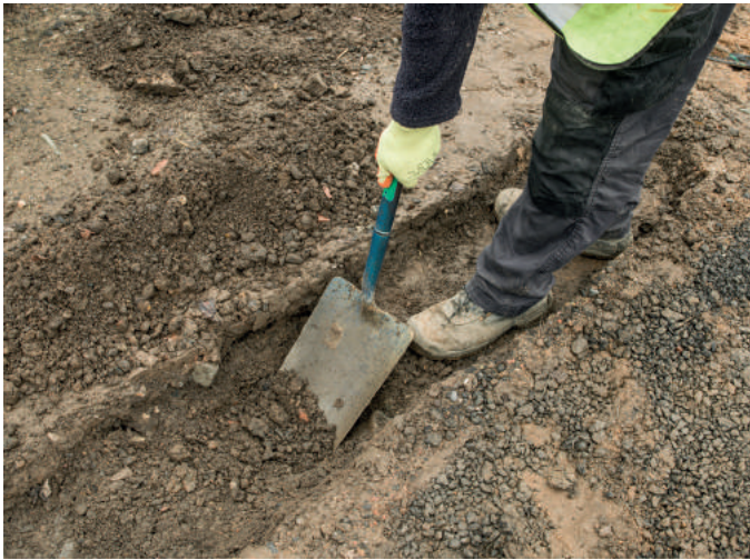
1. Excavate a suitable strip footing to support the Drainer units.
