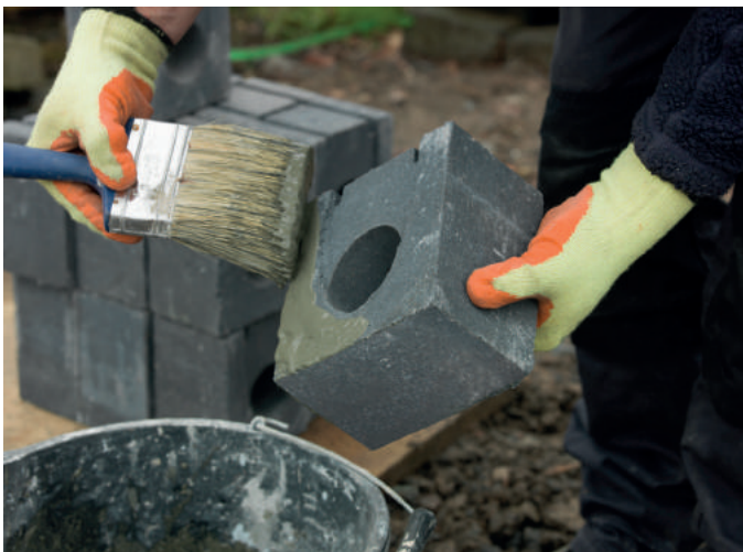
3. Before installing the Drainer units, apply a 5mm bead of M-Flex or paste M-Fix compound from the top of the aperture.
